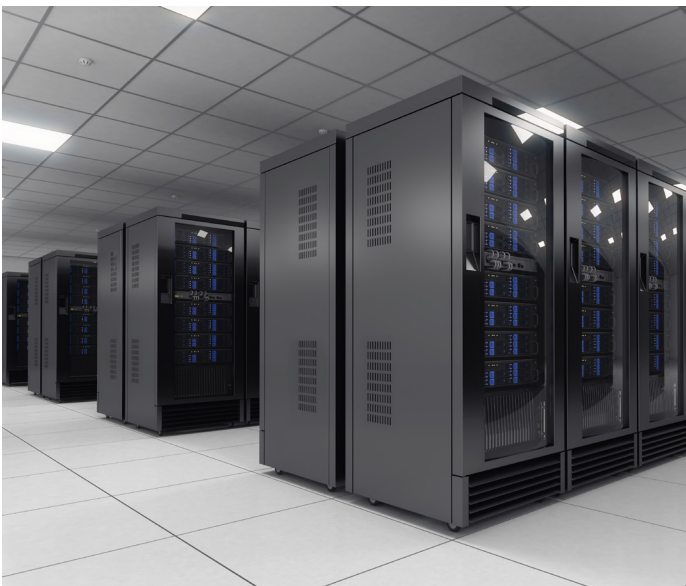
Figure 13: Data hall with an interior suspended ceiling and acoustic ceiling tiles.
