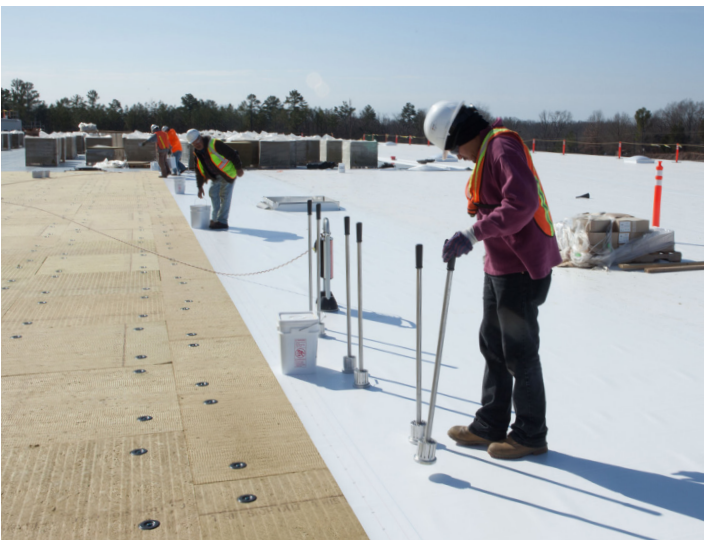
Figure 10: Installation of a PVC KEE single ply roofing membrane over ROCKWOOL Toprock® DD stone wool insulation.
